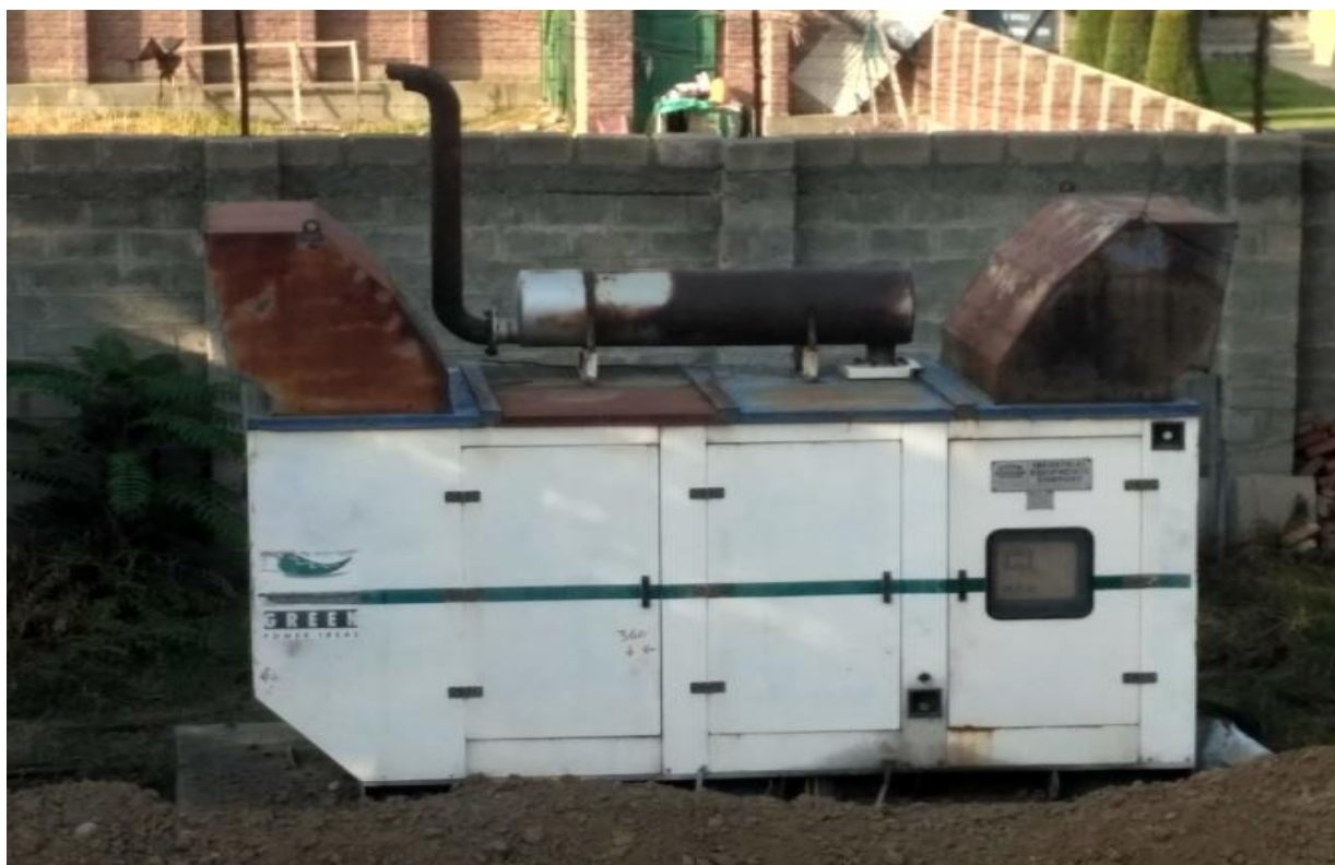
Plate 2. A diesel generator installed near Environmental Science department.
